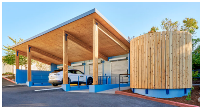
The solar-powered ROSE Port resiliency hub. Photo by Bill Purcell.
