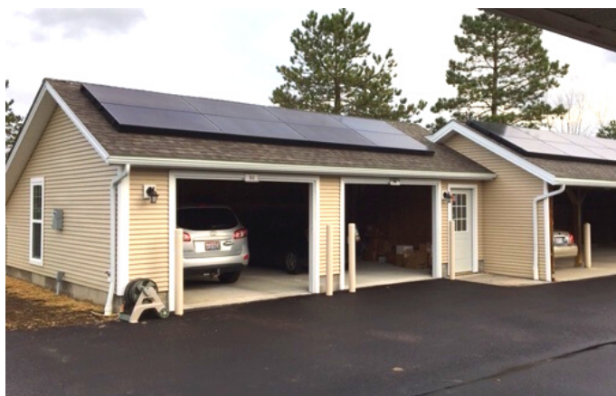
Solar panels on carports at KaO.
