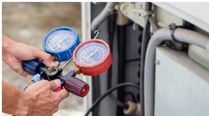
*Service technician using gauges to check refrigerant. Source: Getty Images.*
